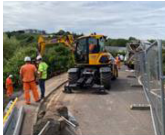
Gabions being filled with rocks adjacent to proposed dev site
