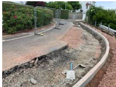
Road being prepared for re tarmac
